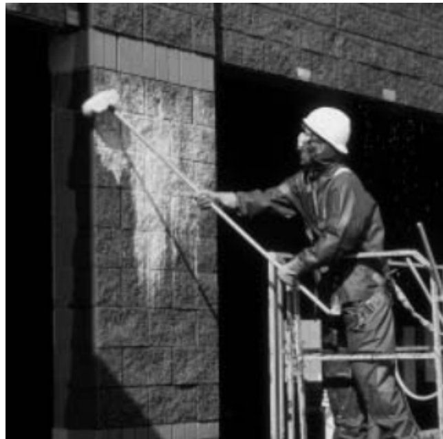
📷 Figure 1—Pressure Chemical Cleaning (photo courtesy of PROSOCO, Inc.)
