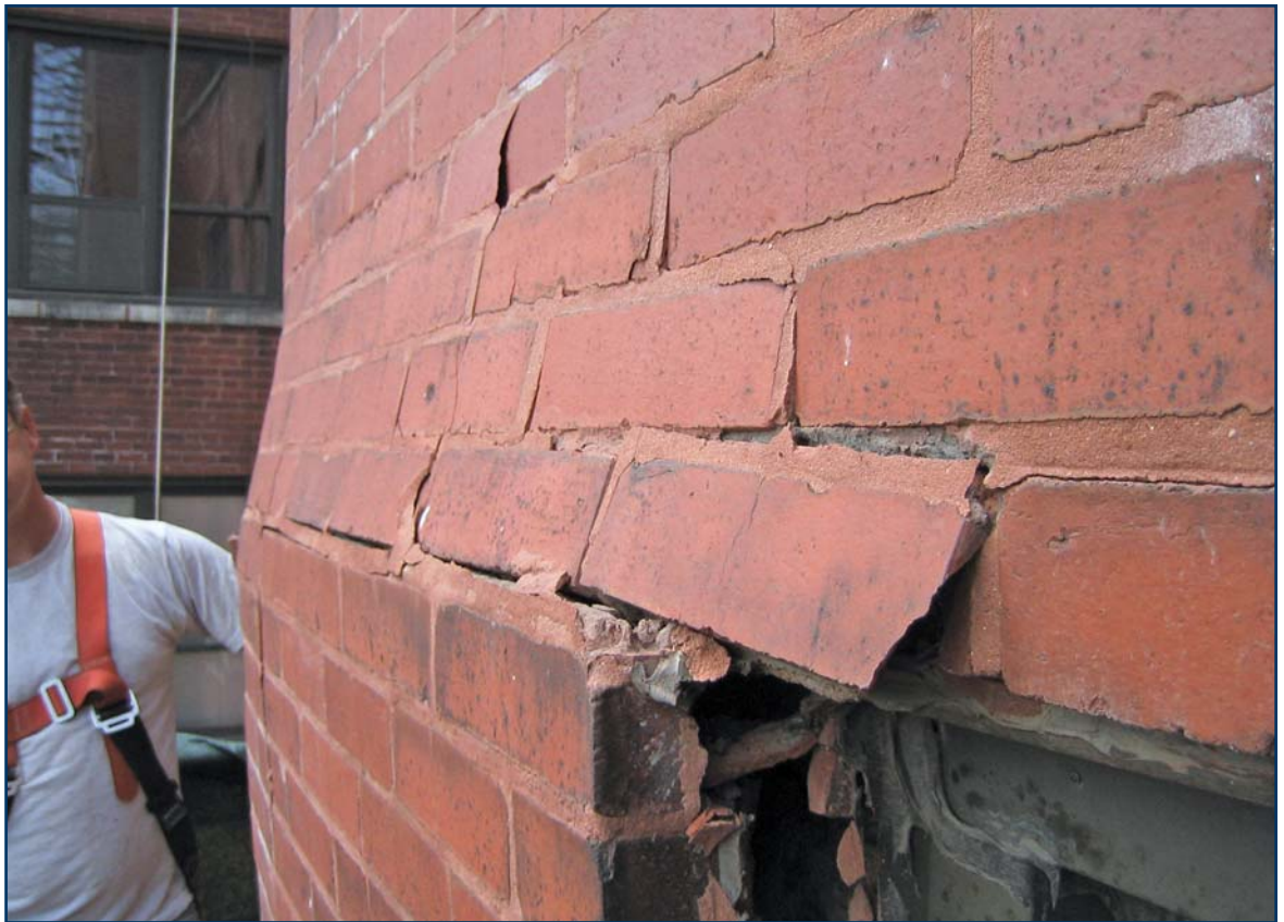
Figure 9 – Displaced brickwork.
