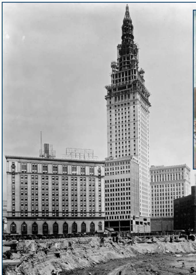
Figure 1 – Skeleton-frame building under construction (image from www.skyscrapercity.com ).
