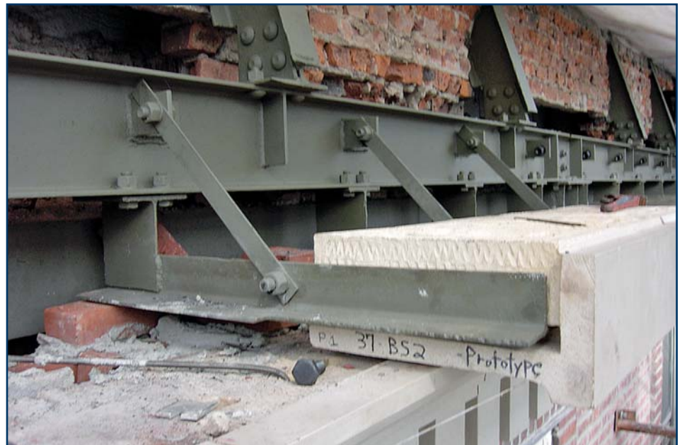
Figure 11 – Coating of existing steel support with corrosion-inhibiting system.
