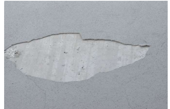
2. Debonding/Delaminating
